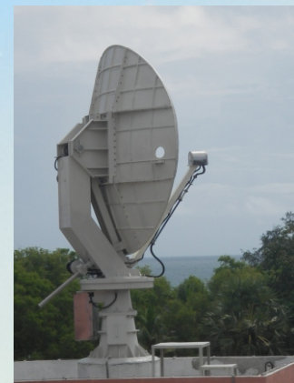
Primary Surveillance Radar
